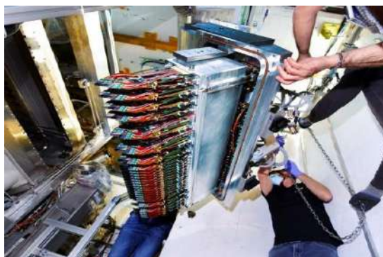
Pictures: (left) Front view of SciFi tracker once installation was completed in spring 2022 and its position carefully adjusted as close as possible (2mm) to the beam pipe. (right) Proposed 13 years ago, the VELO pixel detector installation marks a crucial milestone. The detector is movable and will come closer to the LHC beam than ever before.
