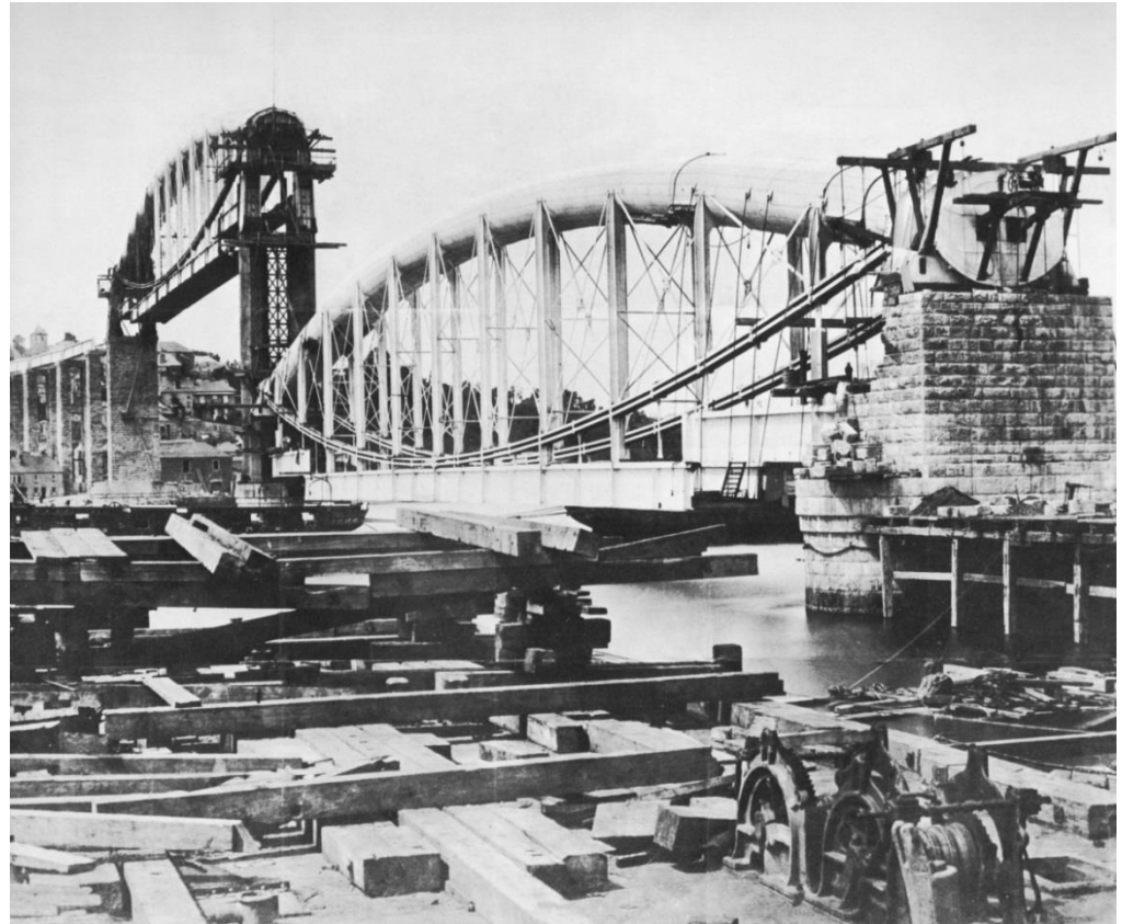
Royal Albert Bridge
